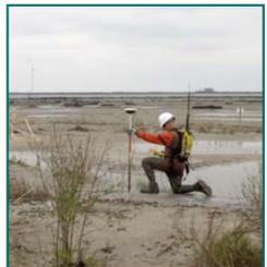
TBS also provided construction bid assistance and construction inspection. The mitigation site was predominantly emergent marsh that converted into a shallow open-water environment. TBS was also responsible for topographic survey and soil borings of both the disposal and dredged areas as well as cross-sections of canals and existing spoil banks.
