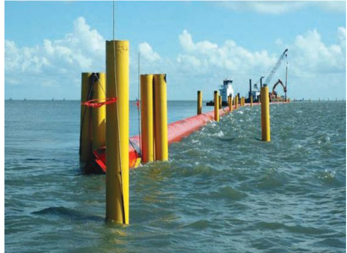
Installation of Rigid Pipe Boom section
