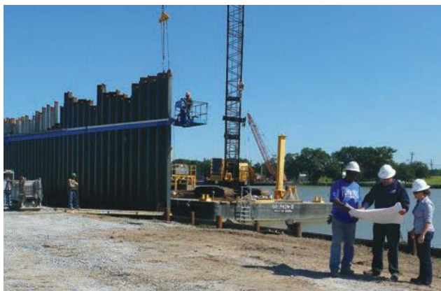
Construction Management - Steel sheetpile bulkhead along the Intracoastal Waterway
