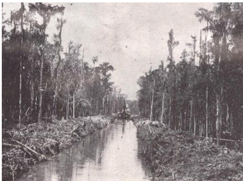
Typical cypress logging canal used to float cypress logs to the cypress mill
