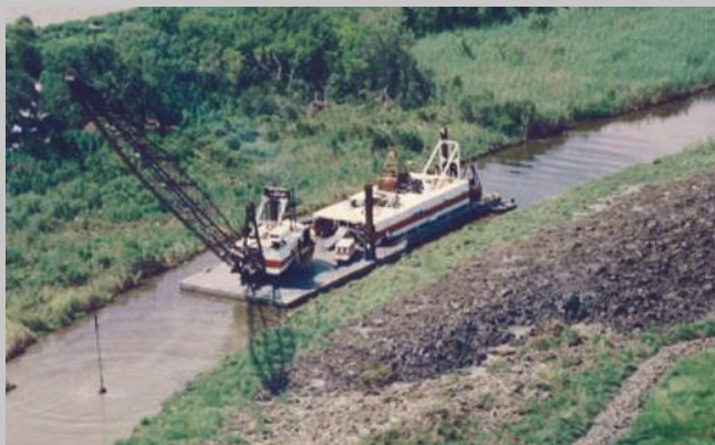
Bayou Terrebonne Levee system under construction - 1990
