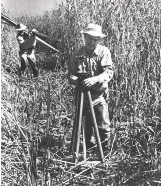
Baker setting up his transit in the marsh for a pipeline survey - 1945
