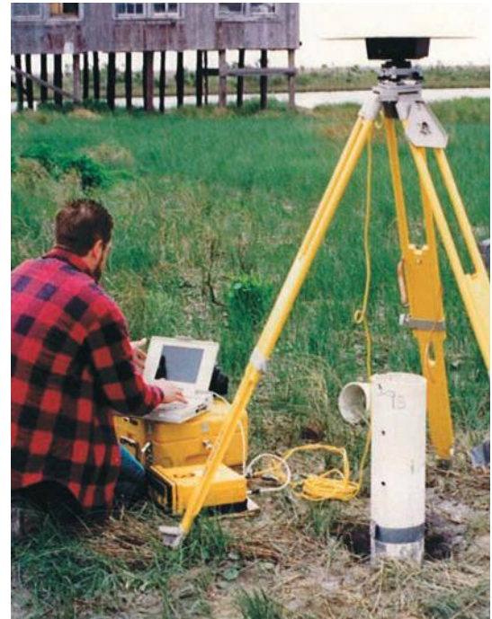
TBS Trimble 4000 GPS receiver on a subsidence survey
