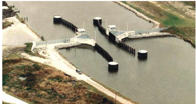
Engineering - Bayou Terrebonne Floodgate
