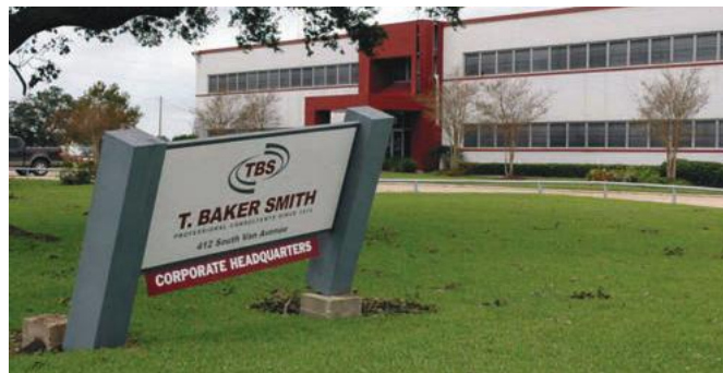
Hurricane Gustav damage to the main TBS facility in Houma - 2008
