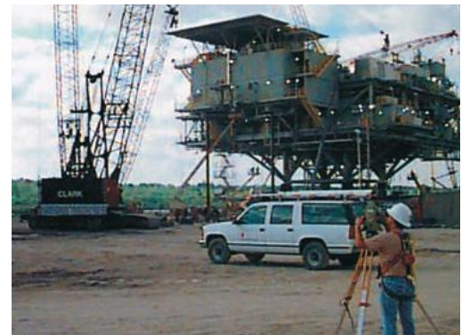
Dimensional Control Survey
