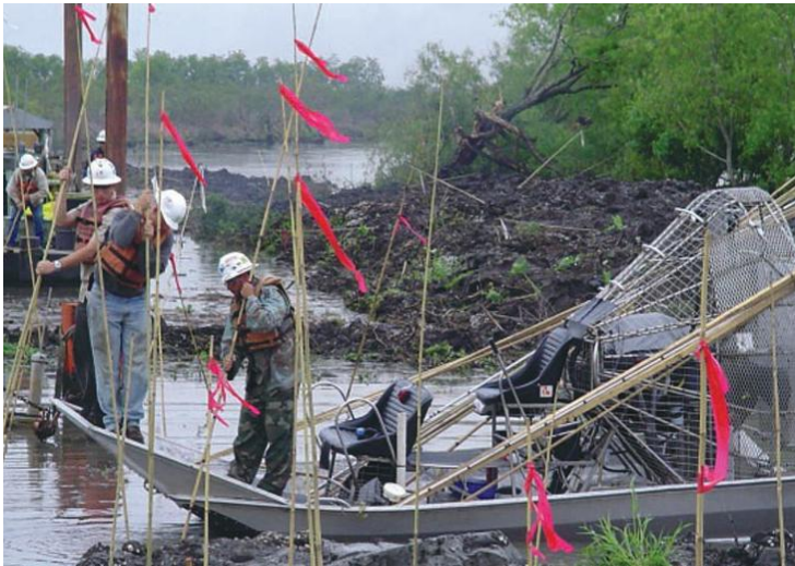
Party Chief Lee Guidry and crew marking a maze of pipelines
