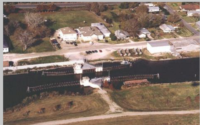
Bayou Petit Caillou floodgate structure - 1988
