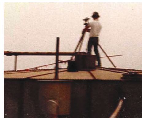
TBS Surveyor setting up his instrument on top of a battery tank at Caillou Island
