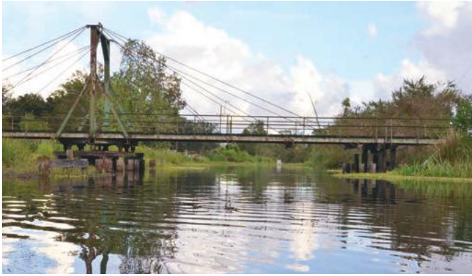
St. Anthony Bridge over Bayou Black, designed by Baker
