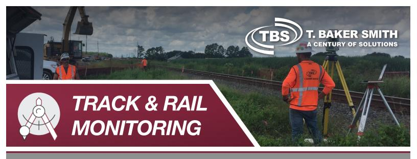
**T. Baker Smith (TBS) leverages dimensional control surveying** methods to monitor track and rail movement. TBS surveyors continuously monitor the track rails for vertical and horizontal movement utilizing highly accurate total station surveying instruments and industrial measurement software to provide real-time dimensional results throughout construction.
