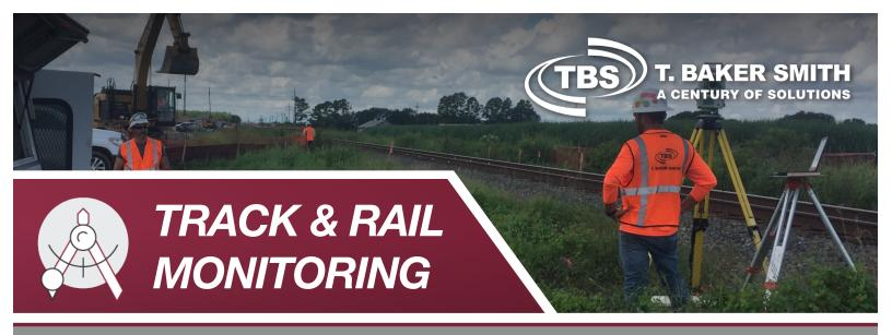
**T. Baker Smith (TBS) leverages dimensional control surveying** methods to monitor track and rail movement. TBS surveyors continuously monitor the track rails for vertical and horizontal movement utilizing highly accurate total station surveying instruments and industrial measurement software to provide real-time dimensional results throughout construction.
